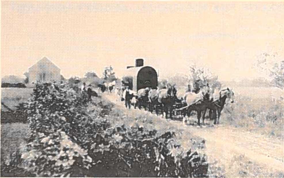
NEW BOILER FOR BRADLEY'S AXE FACTORY. We were given several pictures of the new boiler being hauled to and installed in the axe factory. This picture shows the boiler being hauled by four teams of horses along a road between Westport and the factory site on Lyons Plains road.
