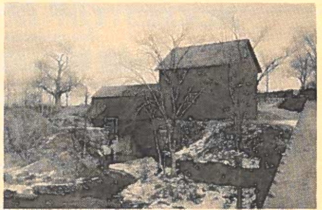
Storehouse. This was used to store lumber that was sawn in the sawmill (the lower building on the left of this building). At one time there was a mill wheel on this side of the building, but, in later years a shaft was run along the top of the dam from the grinding shop on the other side of the dam (from the waterwheel). This building was the subject of our picture quiz last issue. It is now the home of Mr. & Mrs. William Wiehl.
