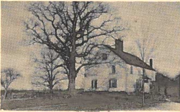
The old David Coley (1715-1802) Homestead. This house was built in the early 1700's and is still standing on River Road. This picture is looking northeast. River Road curves north on the left. The old oak tree has gone, and several changes have been made to the house. The slave quarters on the east side was removed (another addition has been added on since). The large central chimney extends all the way to the cellar, where some of the beams were built into the stone chimney foundation.
