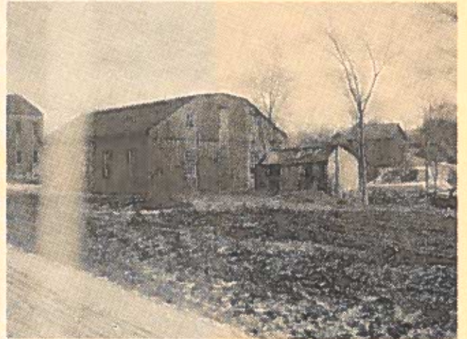
Foundry and tool shed. Iron was melted in the furnace and poured into molds in this building. In the upper right can be seen the store house and River Road. The road in the foreground is Goodhill Rd. The grinding shop and the dam are behind this building.
