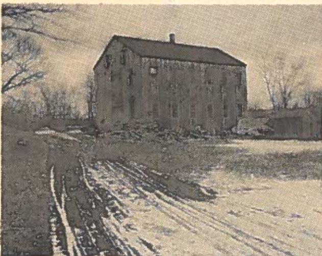
The Machine shop is in background. A shaft ran from the grinding shop to run the milling equipment in this building. The buggy and wagon wheel tracks, highlighted by the snow in the foreground, show where Goodhill Road is located.
