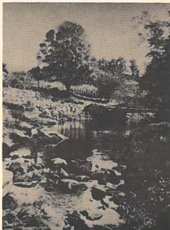
Bridge by Cobb's Mill, looking south. Routes 53 and 57 divide to left of bridge. Mill Pond is beyond bridge.
