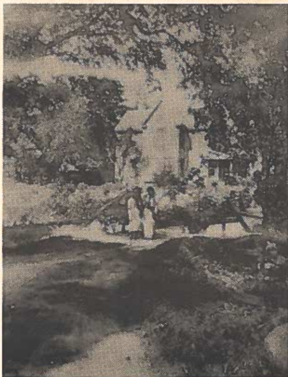
Looking east across the bridge with The Adams Farmhouse in background.
