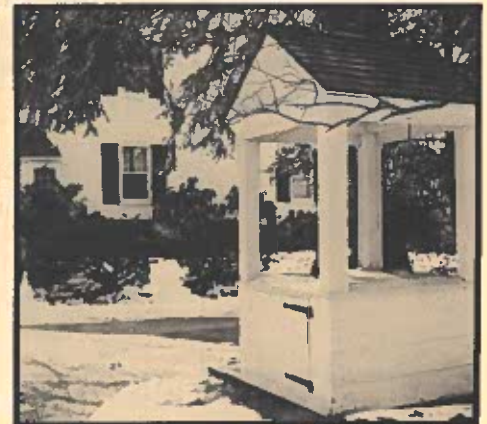
The pump was in the basement of the house on the left and pumped water from the well on the right into a large tank in the basement.
