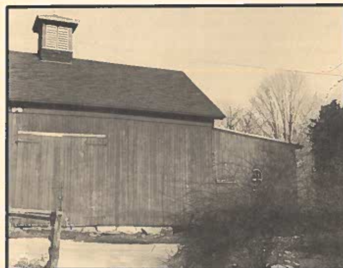
The south side of the barn. Where the shrubs are on the right is where the two story horse barn stood. The horses were on the first floor and hay was kept on the top.
