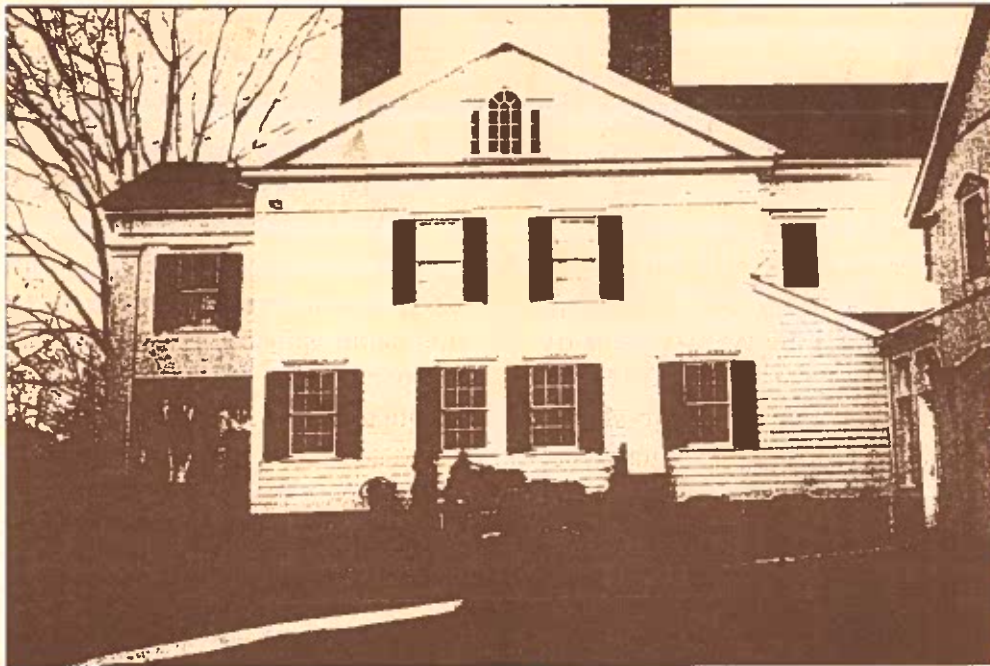
The north face of the original house. The two fireplaces and the placement of windows indicate that the room on the first floor was originally two rooms.
