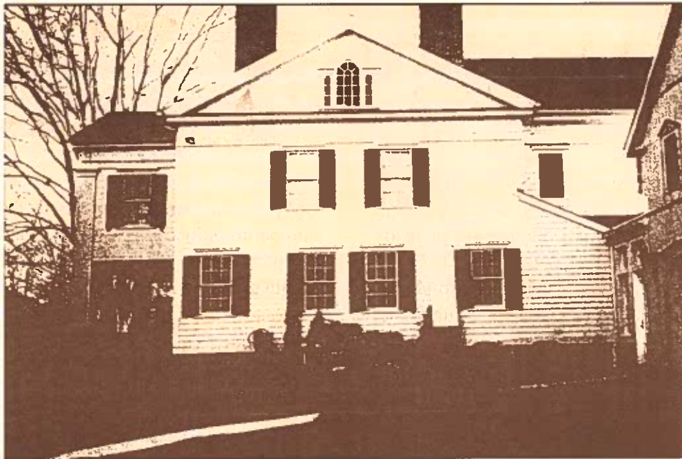
The north face of the original house. The two fireplaces and the placement of windows indicate that the room on the first floor was originally two rooms.
