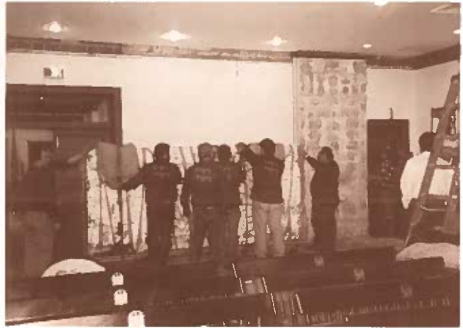
#1 panel in place in town hall
