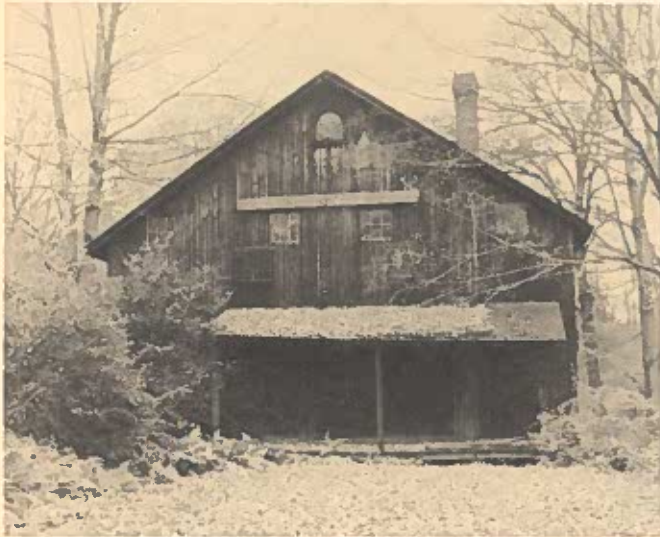
THE WESTON TOY FACTORY BUILDING
