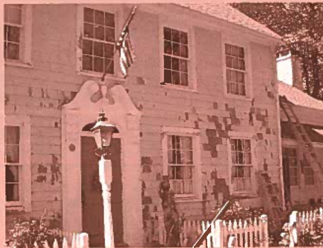
Fixing up the outside for a new coat of paint.
