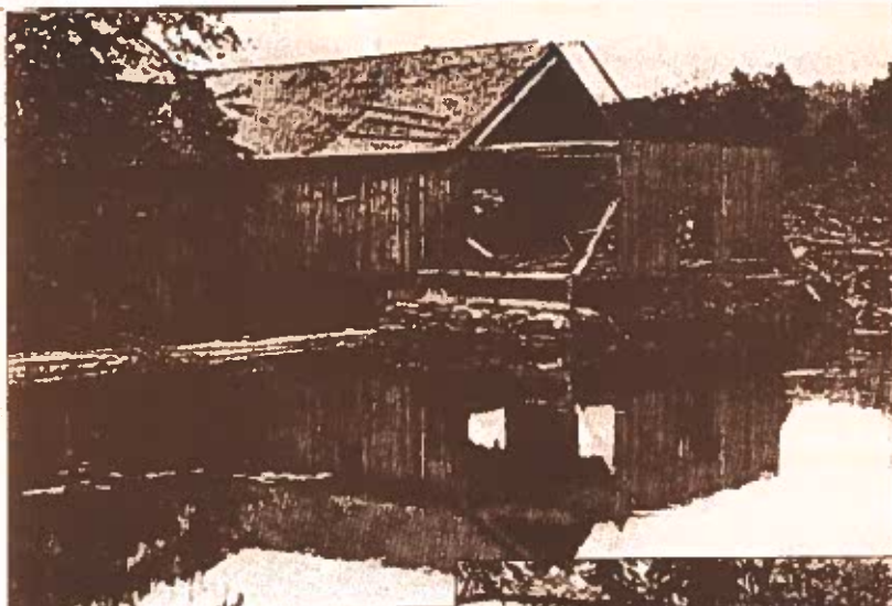
Cobb's Mill Inn (insert), is now a fine restaurant and the only place in this non-commercial town where one may buy a drink at the bar. Years earlier, it was the sawmill and gristmill shown in the larger photo. Located on the Saugatuck, it still boasts the old dam and parts of the original structure.
