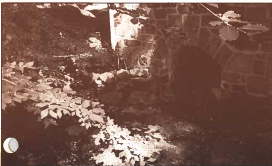
Exit of brook tunnel that runs under the house.
