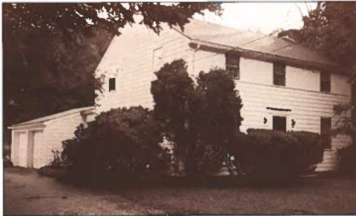
Above: Home of Mary Jungling built by Jim Coley in the 1950's. (The house has black shutters but they were off due to painting.) Below and Right: Jim Coley's contracts and invoices.
