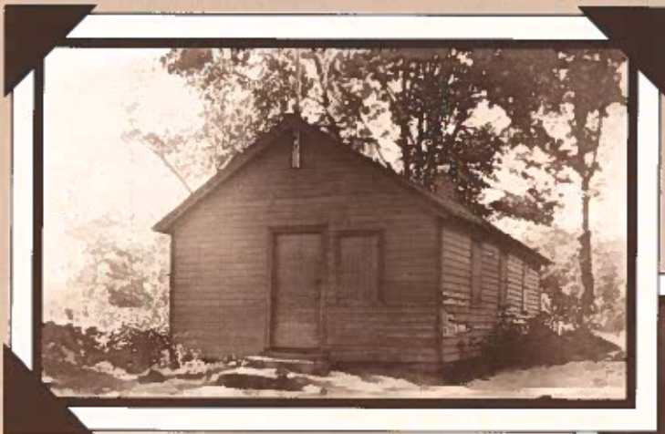
◀ Good Hill Parish School exterior
