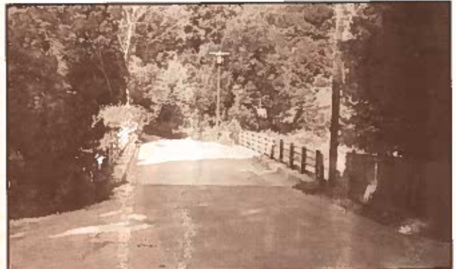
New River Road Bridge
