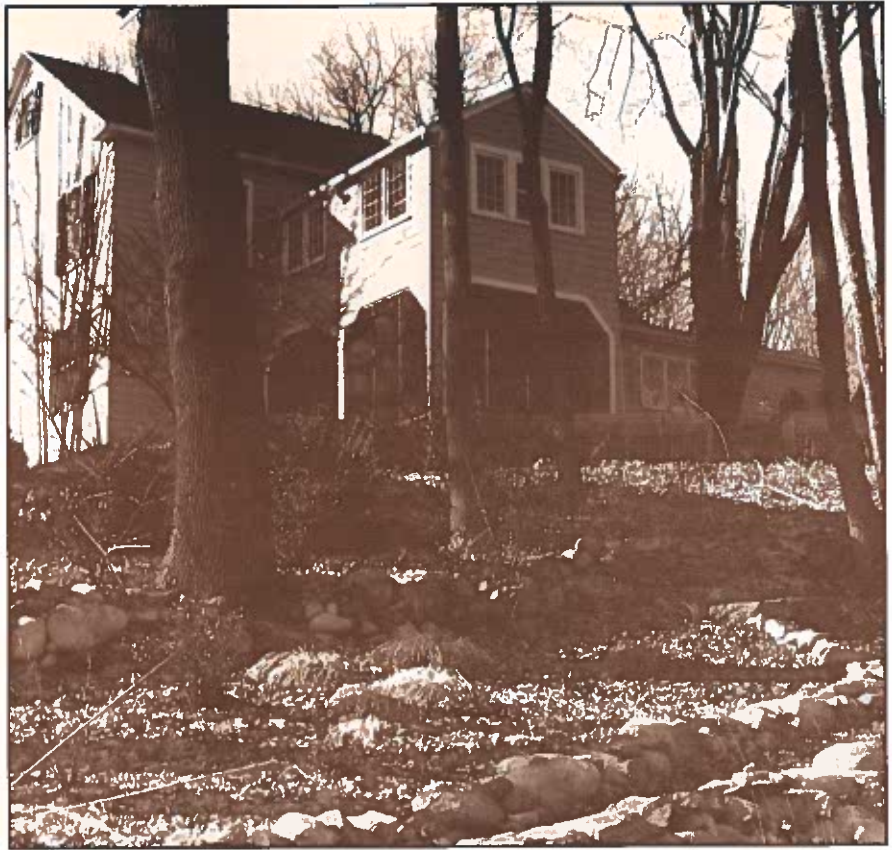
The backyard of One River Road belonging to Alan and Myra Aronow. Myra has been rebuilding the stone walls and designing the gardens.
