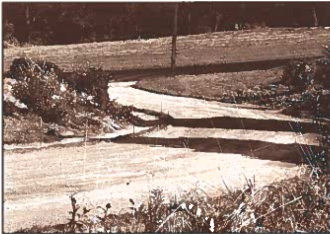
Preparation work for paving the driveway at the Coley house coordinated by Joe Spetly.
