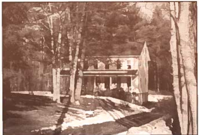
Ebenezer Morehouse House - 1861, now owned by Ernest Albin, a descendent. The house was moved from across the road in 1960 just before Mr. and Mrs. Albin moved in.
