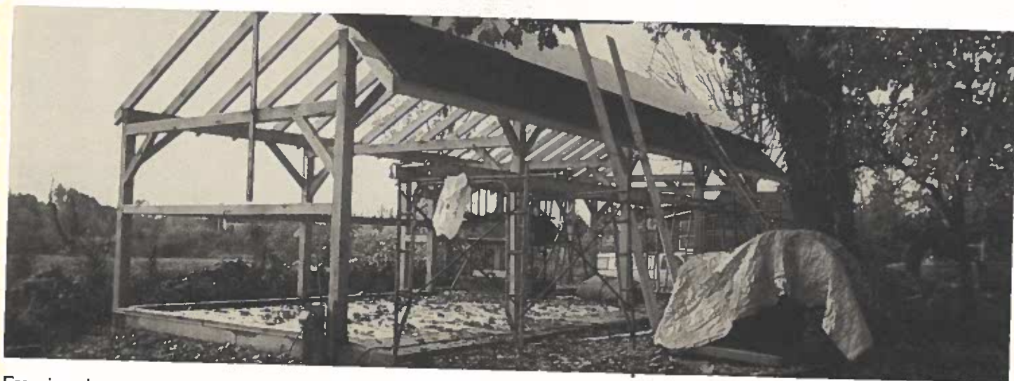
Framing done—putting on the roof.
