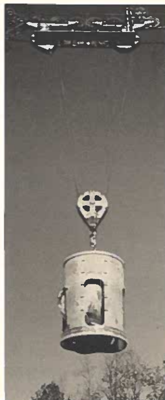
Concrete bucket moving on cable to Saugatuck Dam site.
